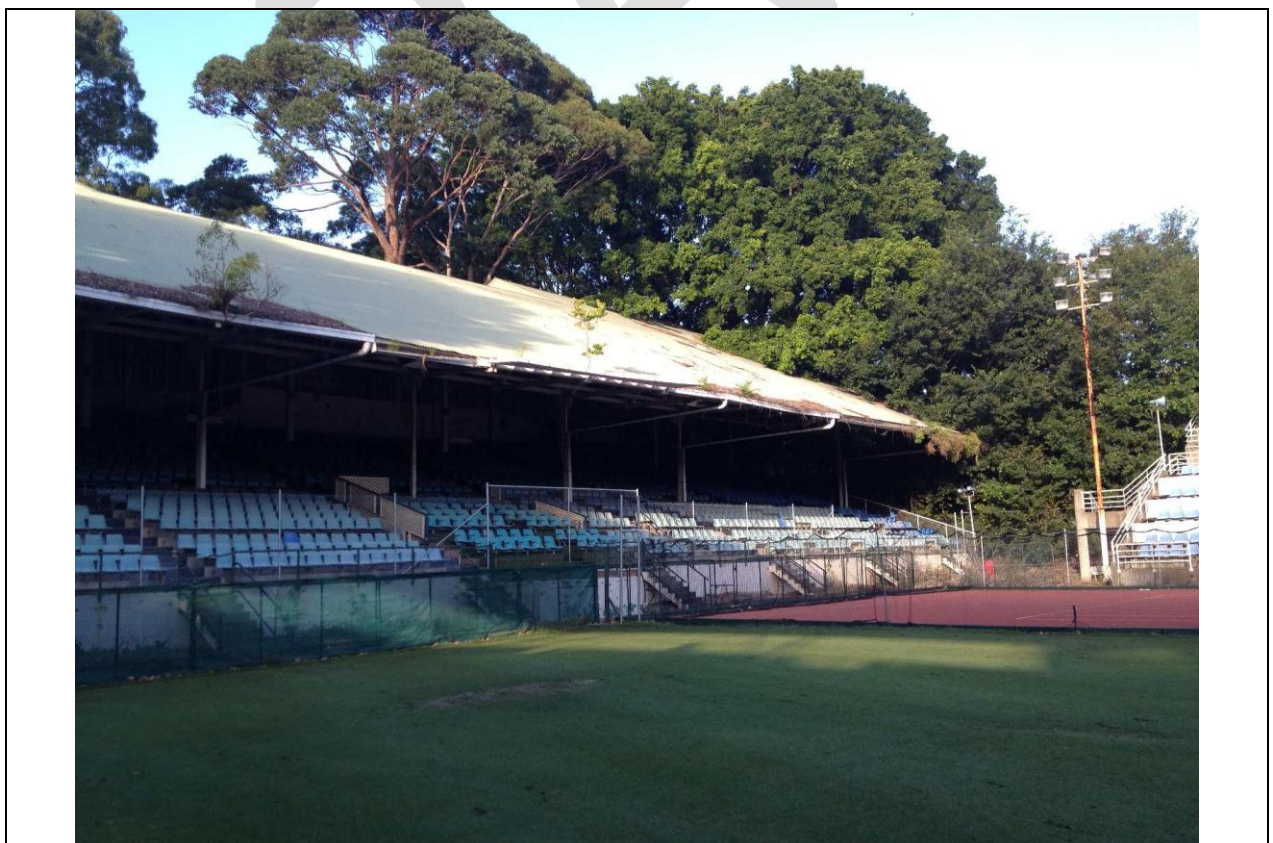
The southern grandstand looking southwest – view of roof scale, vegetated backdrop
