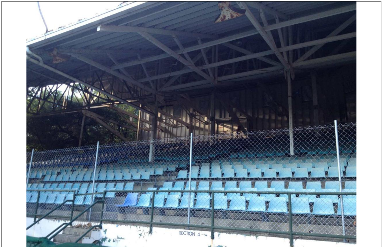
The southern grandstand looking southeast showing the complex superstructure and later steel truss additions
