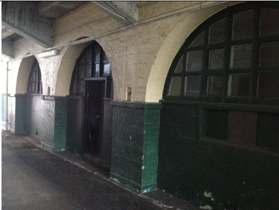
The Marsh Stand structure with infill joinery and traditional paint scheme
